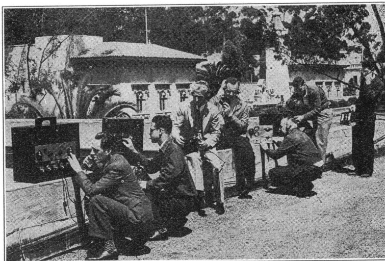
This gang worked three days making a transmitting and reception survey in connection with the Radio Amateur Fiesta, July 20, 21.
