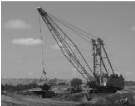
Fig. 13b. Loading equipment too large for truck.
